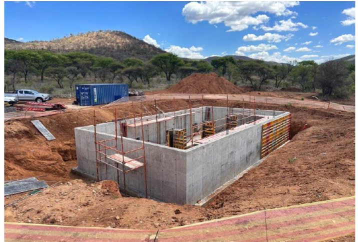
Pump Station 1 Concrete to Walls & Columns
